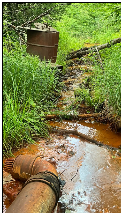
A permanent chemical treatment line is attached to the deep mine's wet seal discharge pipe that drains to the headwaters of the South Fork Cherry River. (West Virginia Department of Environmental Protection)
